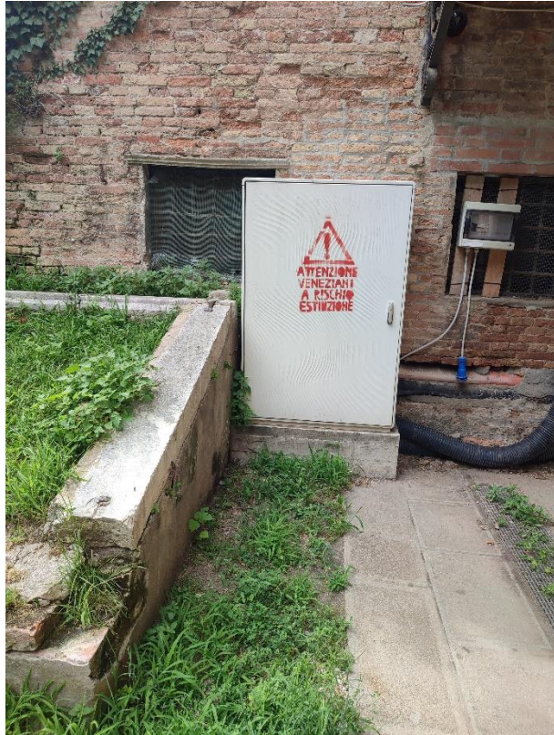
Fig. 9: Risk of extinction for Venetians.
