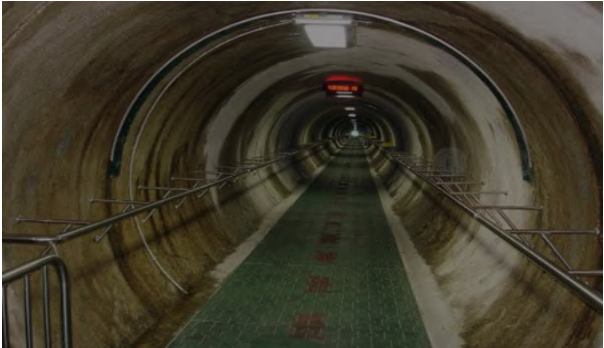
Figure 19. The third infiltration tunnel.
