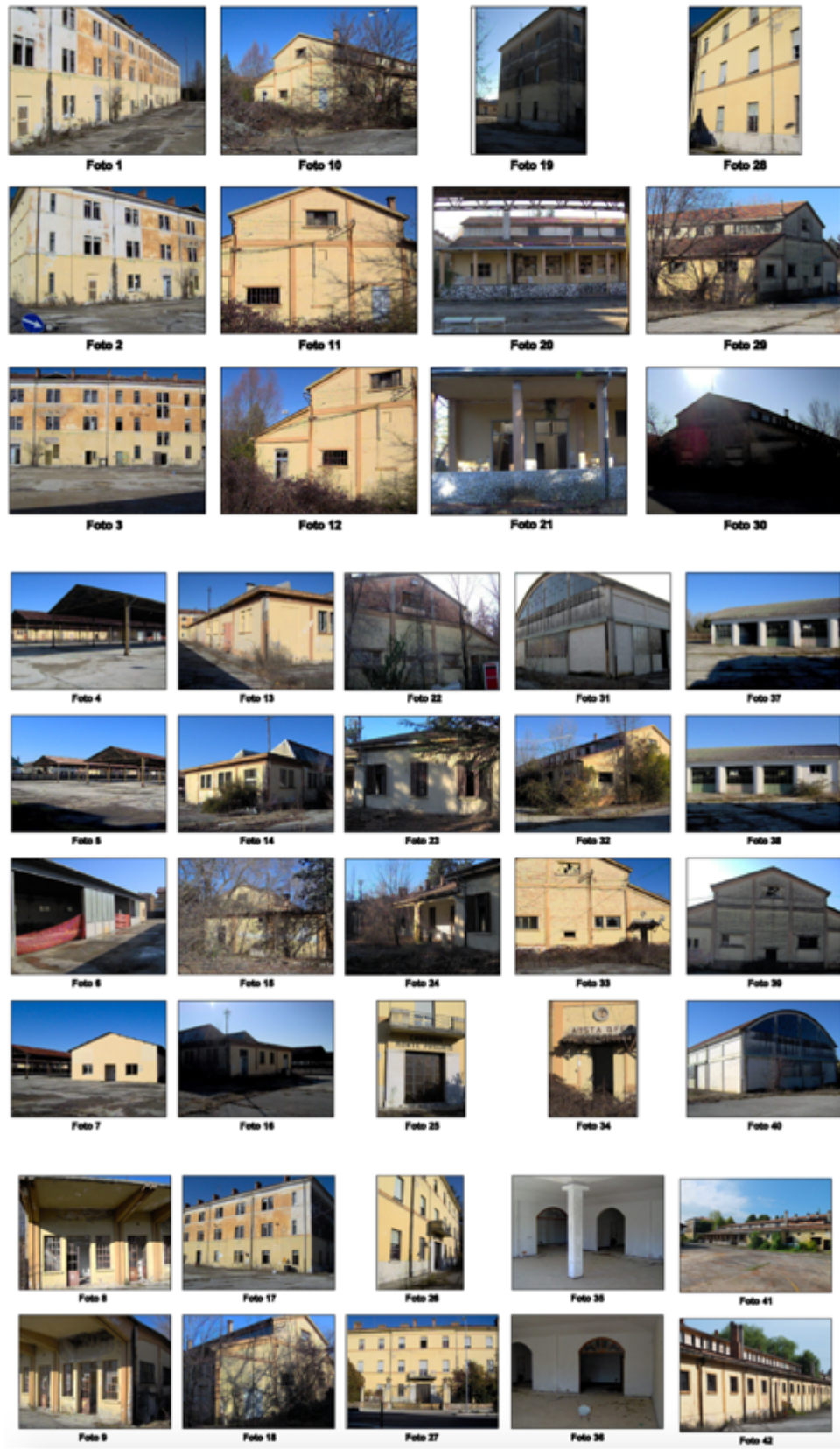
Figure 5.2: Current situation of the barracks
