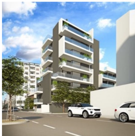
Figure 5.10: Example of a green condominium that will be realized in Mestre (VE)
