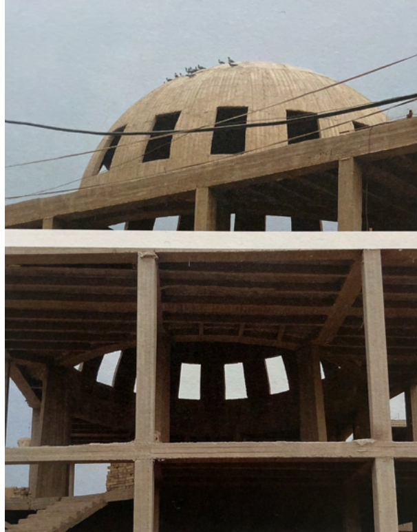
Figure 27: The private museum by Hussein Harba under construction. Before 2013. Schroth, 2013, p.19.
