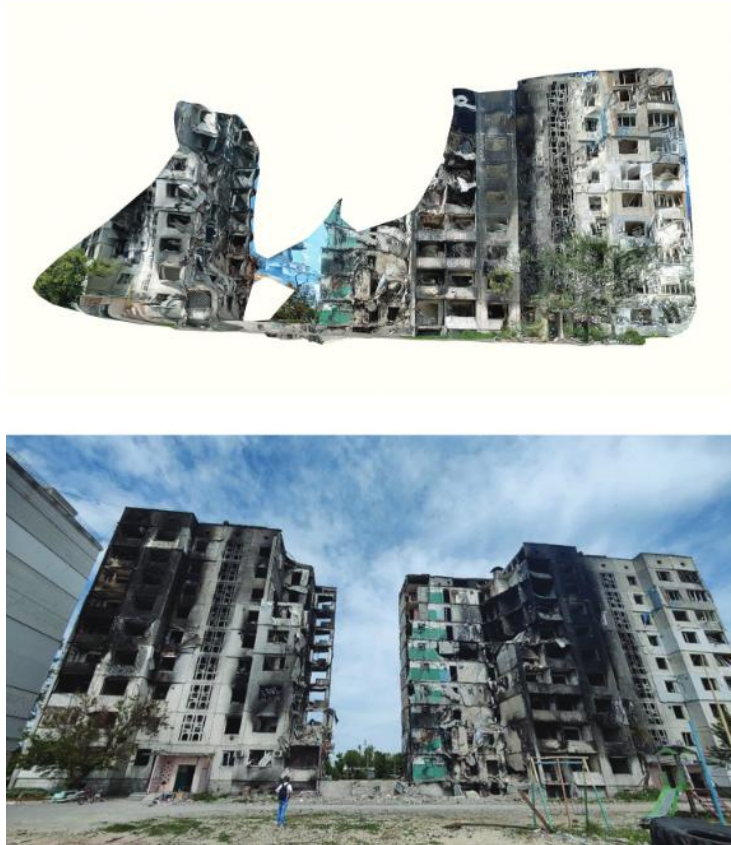
Figure 19. – Standard photograph and 3d scan generated using the polycam app by MaximKamynin of burntout residential buildings in Borodyanka, Ukraine. ©TBA - Maxim Kamynin &CNN. All backup Ukraine archive is under creative commons 4.4 Attribution.
