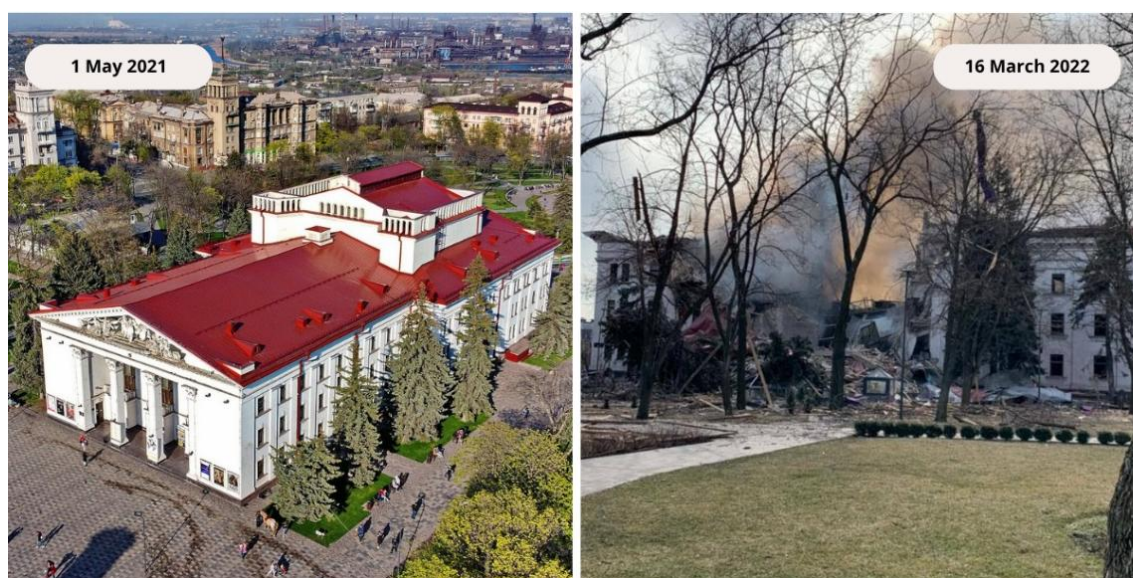
Figure 16 – Donetsk Academic Regional Drama Theatre, Mariupol, before and after the attack of 16 March 2022. Left: pre-war aerial view, 1 May 2021, photograph by Oleksandr Malyon. Right: damage documented on 16 March 2022, photograph by the Donetsk Regional Military Administration. Licensed under CC BY-SA 4.0.
