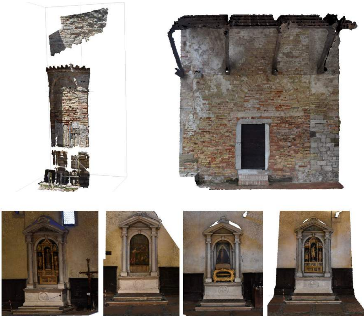
42 Upper left: the model of the outer smaller crypt apse; Upper right: norther portal; below: the 4 altars from the side naves
