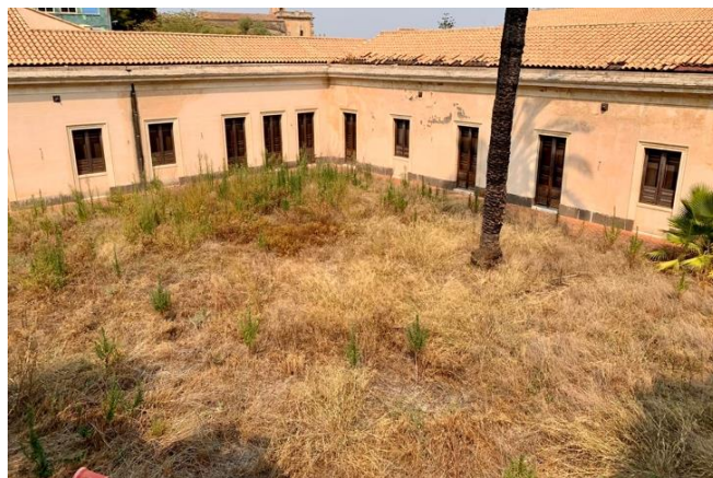
Ill.20 Upper Courtyard and Noble Floor (August 2023)
