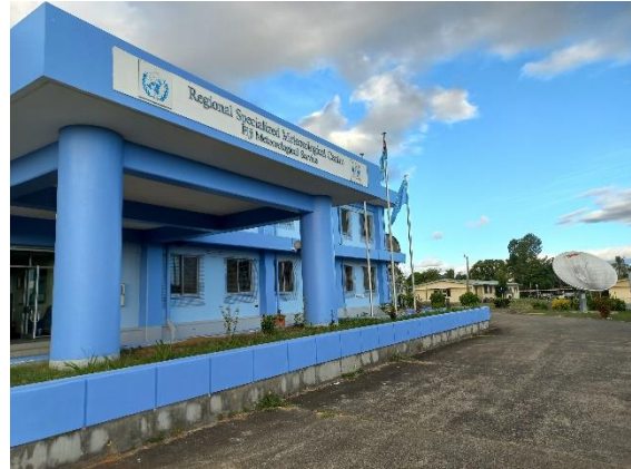
Figure 8. Fiji Meteorological Office, Nadi.
