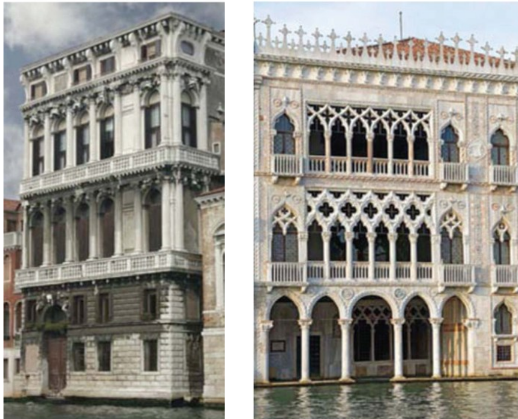
Figure 2- The effects of local pollutants on Flogini's palace and the facade of Ca' d'Oro, in the Grand Canal. The latter shows the original white-stone aspect of historical buildings (Morandin et al., 2015)
